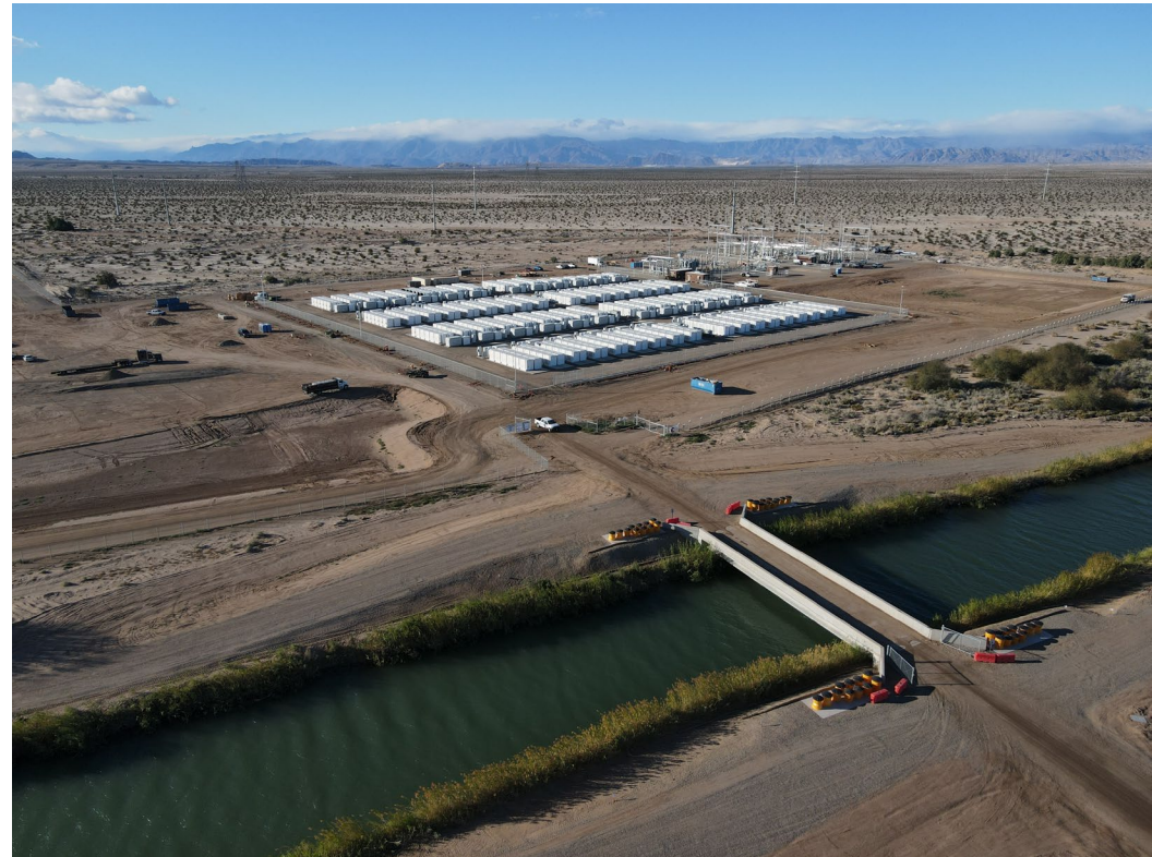
Westside Canal Project, 131 MW, SDG&E, Imperial Valley
